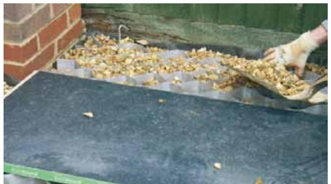
**IMPORTANT : Only crushed, angular infill must be used to fill the cells.**
